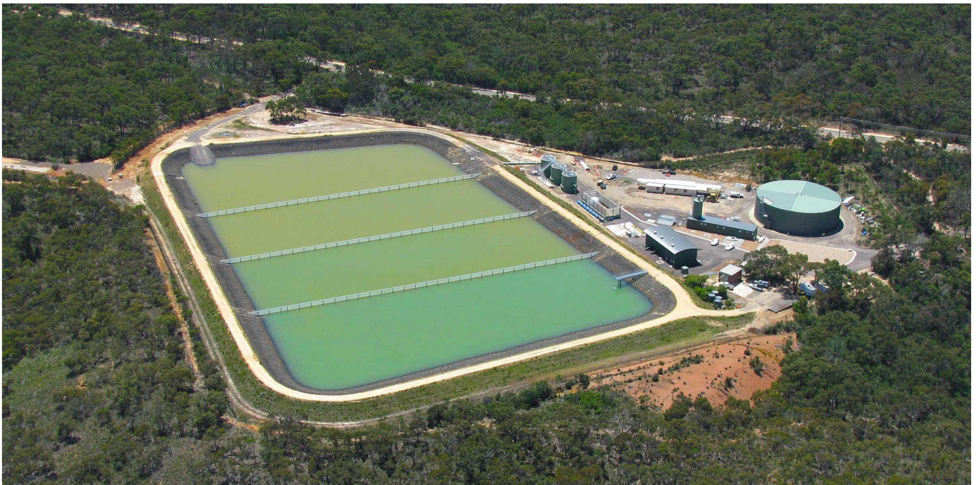
Anglesea borefield pre-treatment plant
