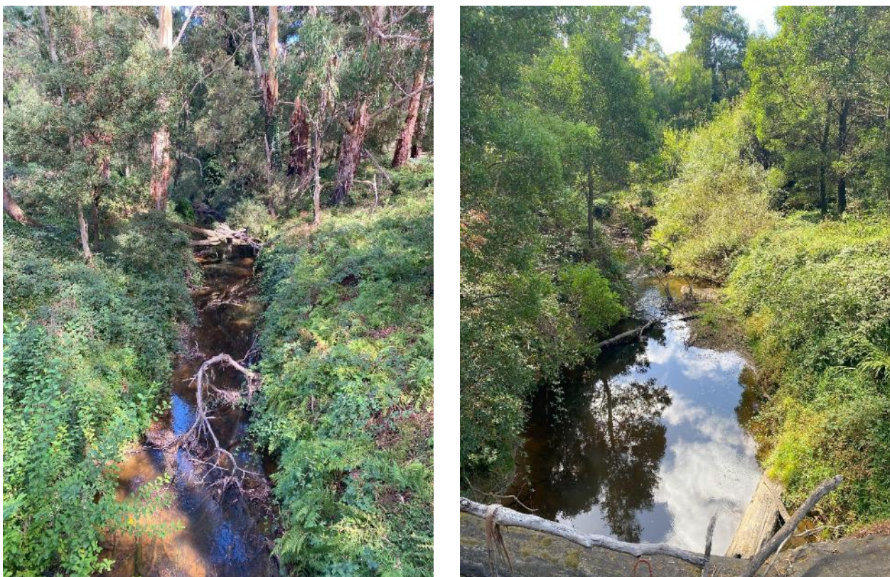
Figure 13. Reach 2a existing site at James Access bridge (Left) looking upstream (right) looking downstream. Image taken 24 March 2025.
