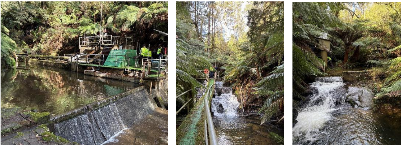
Figure 28. Arkins Creek West branch weirs (left) lower weir (centre) middle weir (right) upper weir. Images taken 21/07/2025 J Bolden.
