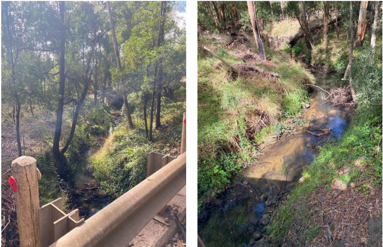
Figure 10. Love Creek at Wonga Road bridge crossing (left) looking upstream (right) looking downstream. Image taken 24 March 2025
