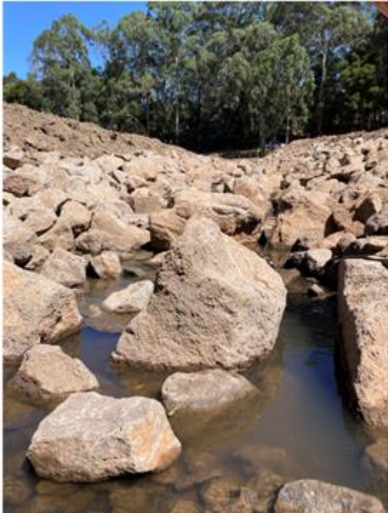
Figure 2: One of the grade control structures installed in the East Barwon River as part of the East Barwon Willow Removal and Restoration Project.
