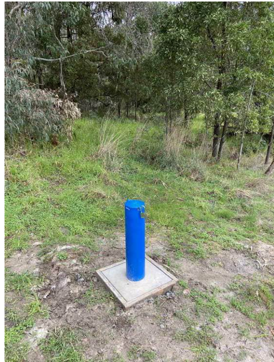
PCBH01V and PCBH02V installed in the same borehole
