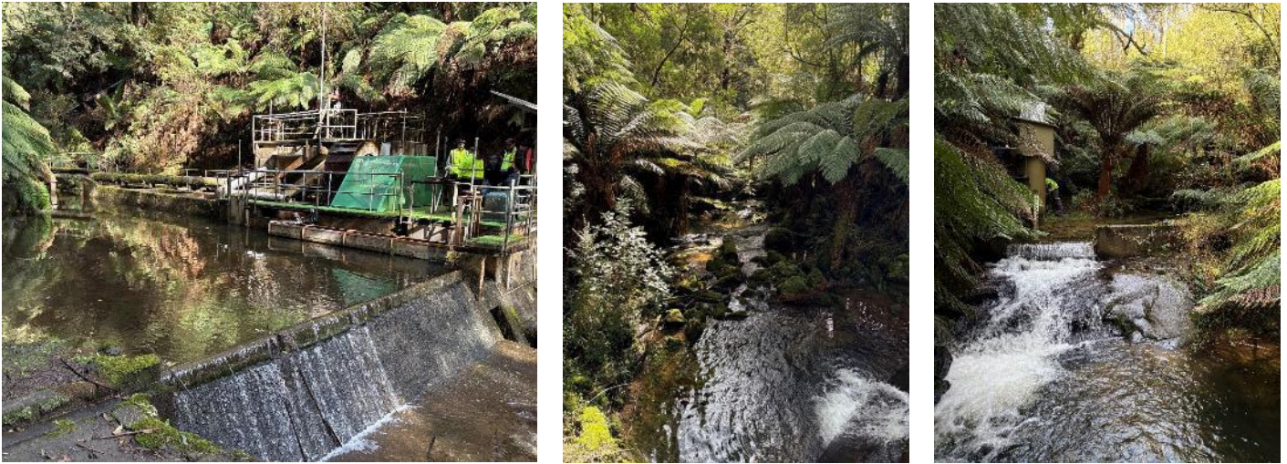
Figure 13. Arkins Creek West Branch (left) lower weir (centre) downstream of bridge (right) upper weir. Images taken 21 July 2025.
